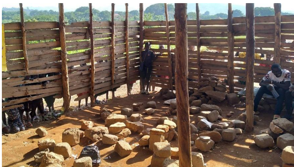
Figure 5: Temporary, makeshift space being used for some voluntary literacy classes in Uganda, while a new building is under construction.
