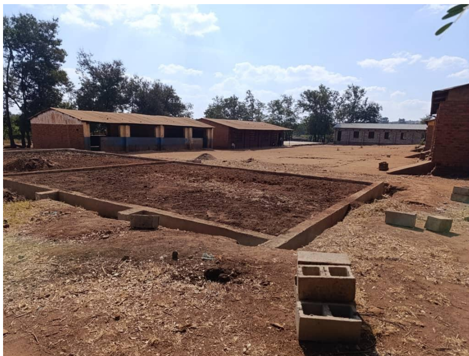
Figure 4: foundations for new classrooms at Chibanzi primary school in Malawi
