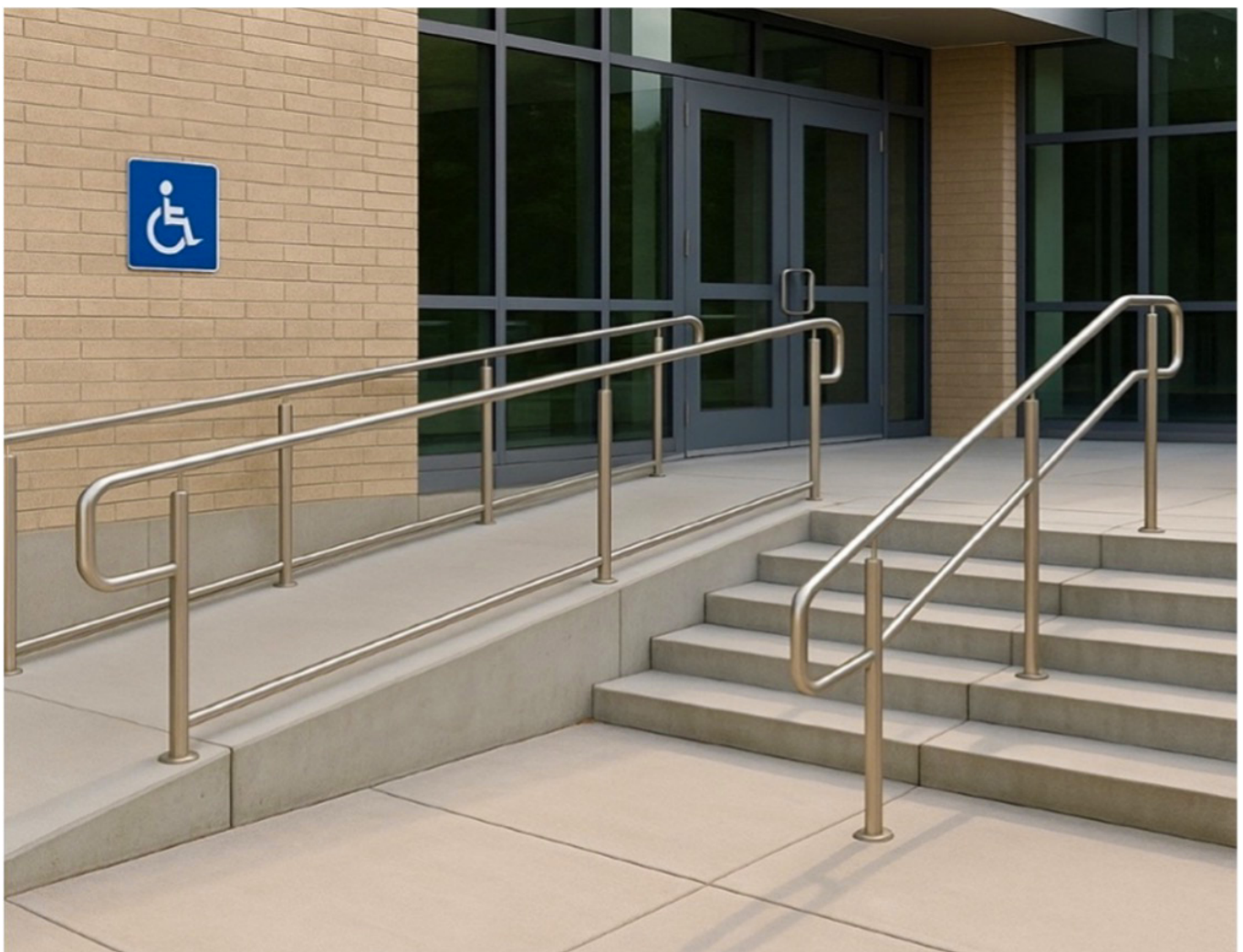
FIGURE 8. Stairs with ramp and handrails (Source: https://www.acumen-studeos.com/ramps-staircases-public-buildings-design/ )
